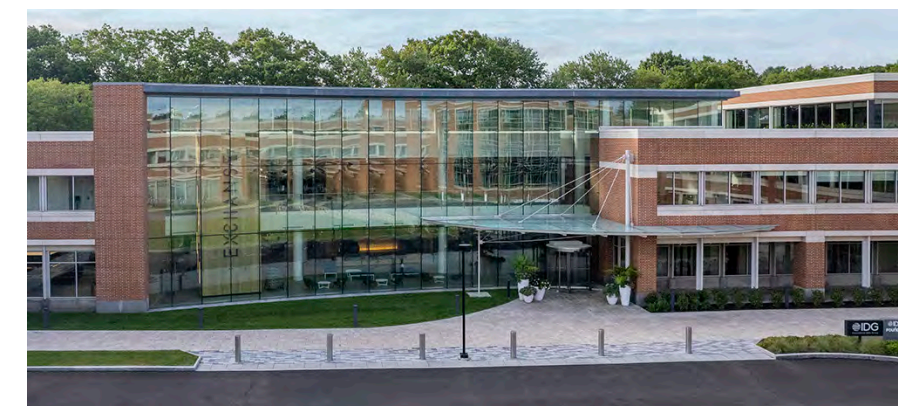
Building A exemplifies a high performance workplace reflected in LEED Gold certification and LEED Zero Carbon project targets.
