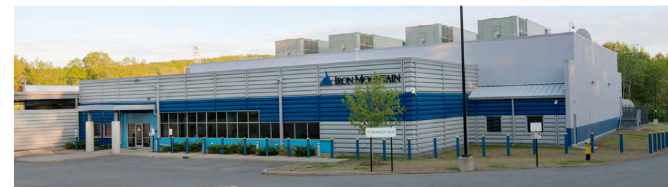
An Iron Mountain data center located in Boston.
