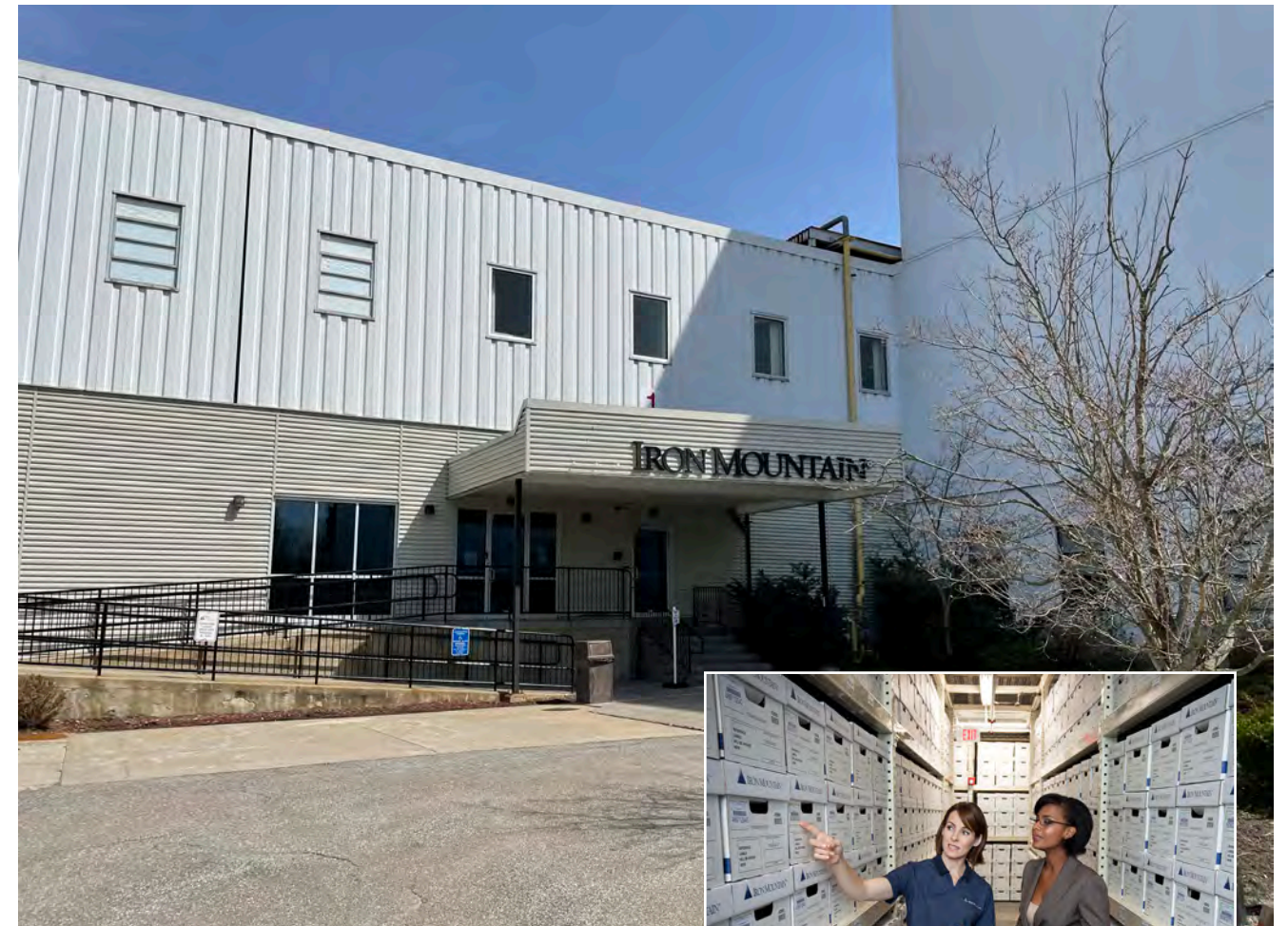
Iron Mountain has thousands of local facilities, including in Northborough, Massachusetts (top), that enable it to respond quickly and maintain flexible services tailored to meet the specific needs of its clients.
